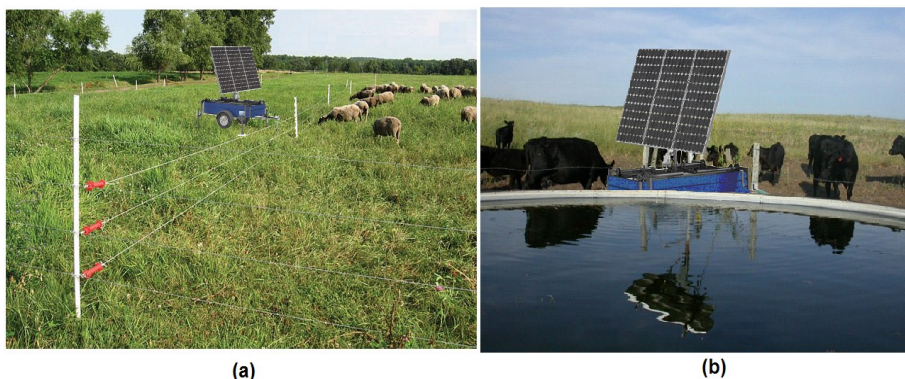
Fig. 23. Possible variants of applications MSG in livestock breeding; (a) mobile solar “electric shepherd”, (b) mobile solar station for watering livestock
