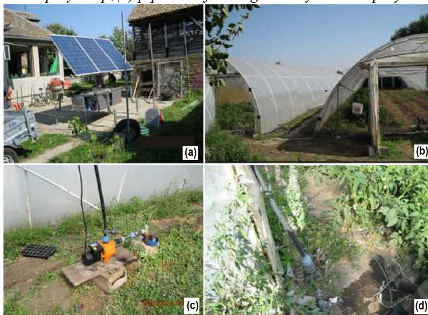
Fig. 22. Application MSG in location village-Veliko Selo; (a) in the courtyard of agricultural households;(b) greenhouses with garden tomatoes; (c) Villager 1500W garden pump connected to the irrigation system drop-by-drop;(d) pipe lines for irrigation system drop-by-drop
